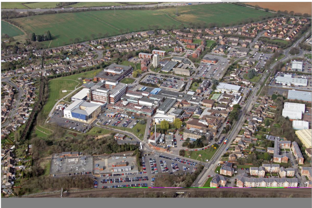
Kettering General Hospital, Rothwell Road, Kettering
